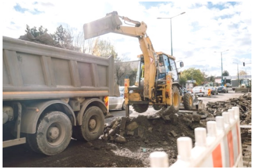
Fig. 9. Excavation operations (own source)
