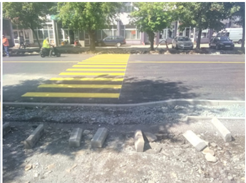
Fig. 5. Street improvement, decking and cladding (own source)
