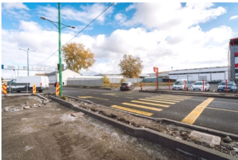
Fig. 10. Street improvement, decking and cladding (own source)
