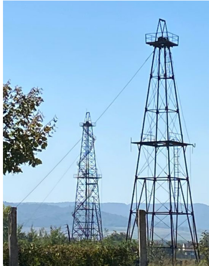
Fig. 3. The salt exploitation wells
