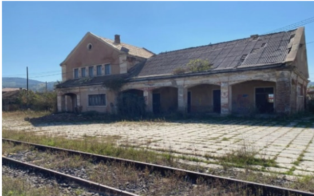
Fig. 5. Building of the station
