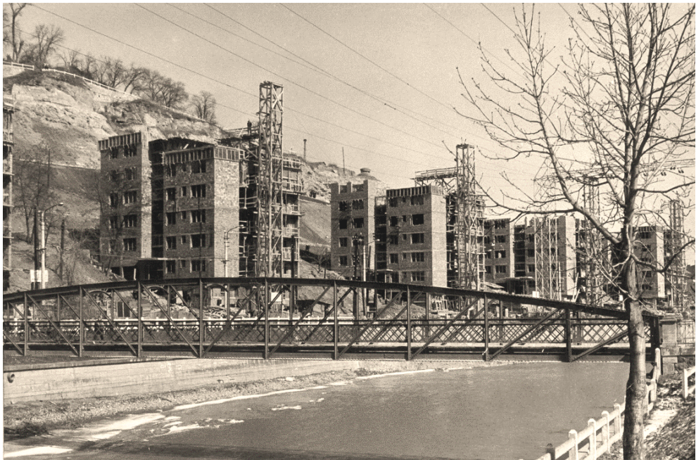
Fig. 10. The slope of the Fortress Hill and the presence of modern blocks of flats at the foot of the hill between 1960 and 1964
