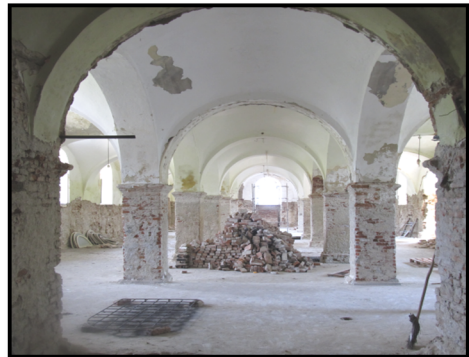
Fig.4. Inner image of D building
