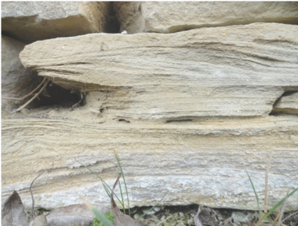
Fig. 4. Delamination and granular disintegration.
