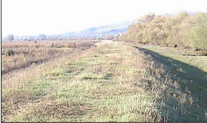
Fig. 1. Dyke on Someșul Mic River, Cetan village (September 2008).
