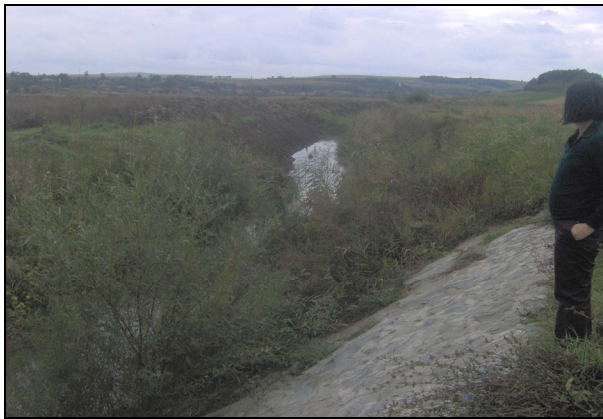
Fig. 4. Cleaning works by removing the natural vegetation on Lujerdiu River (September 2008).
