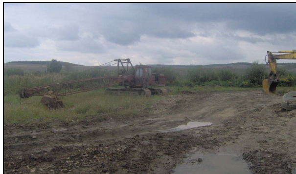
Fig. 6. Correction works on Valea Mărului (September 2008)
