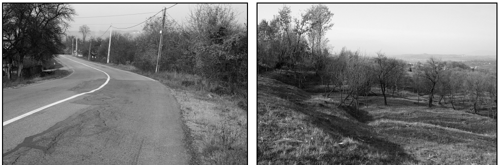
Fig. 10. The road DN 18B from Baia Mare to Tg. Lăpuș (left) and recent landslide movement indicated by tilted young trees in Cărbunari area (2012).
